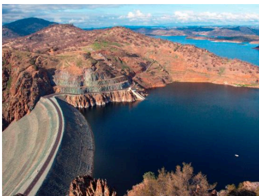
New Melones Dam in California is one of the facilities that will receive funding. They will receive $19.7 million for work in its powerplant.
