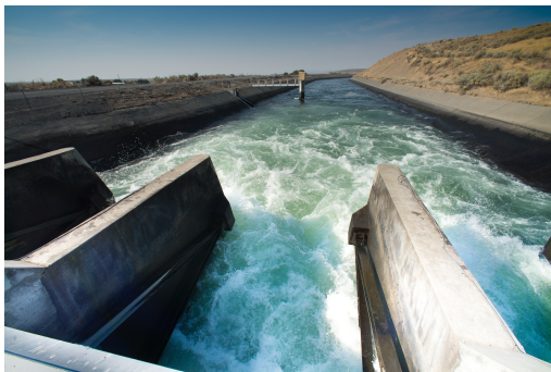
Small projects like gate modernization and meters are examples of projects funded by the Small-Scale Water Efficiency Program.
