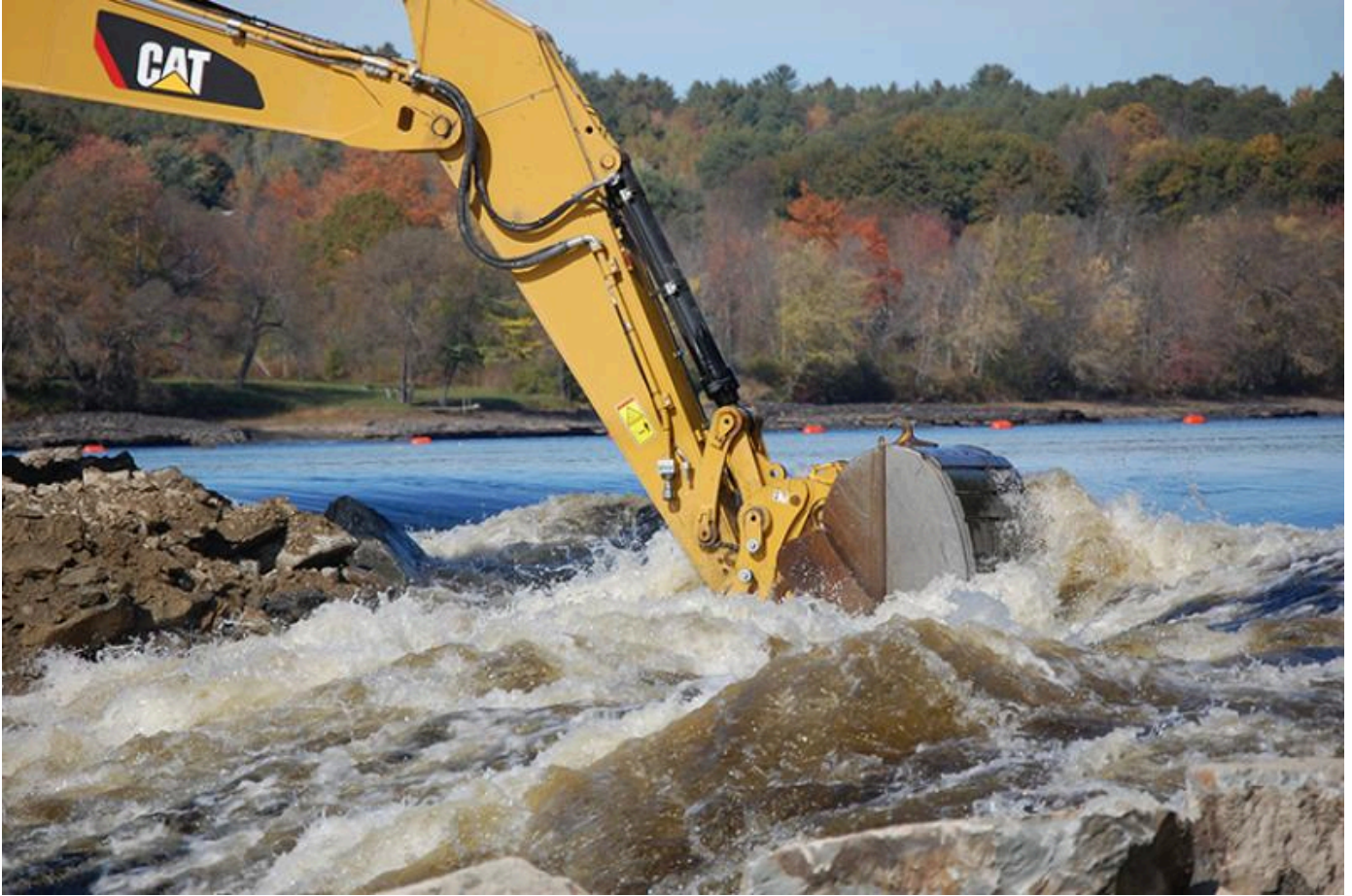
Dam removal on the Penobscot River in Maine. Credit: Penobscot River Restoration Trust.
