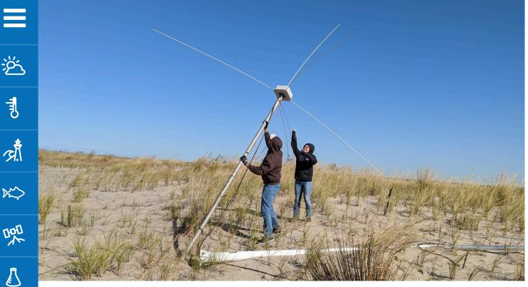
udents from Rutgers University's Masters in Operational Oceanography program installing a highquency radar antenna at Sandy Hook, NJ. This radar is part of the national high-frequency radar twork in the MARACOOS region. There are more than 165 HFRs like this across the U.S., some of hich are more than 24 years old. A portion of the funds from these awards will be used to update, grade, and modernize these critical observing assets. (Image credit: Hugh Roarty, Rutgers University.)
