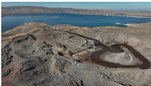
Construction at B.F. Sisk Dam.
