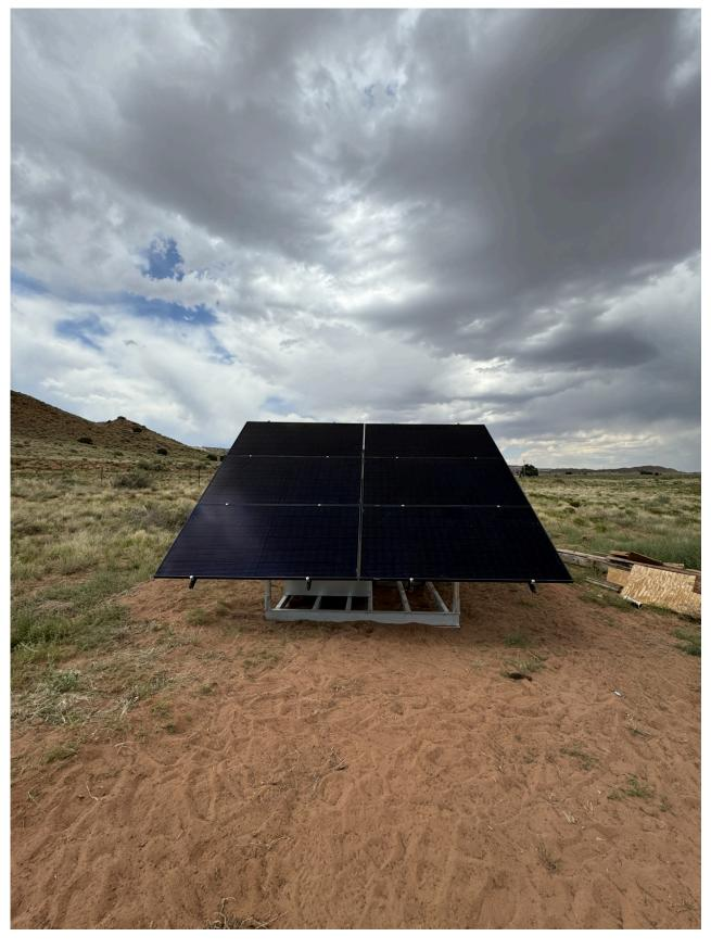
A complete NRI off-grid solar unit with six modules and eight batteries installed on Navajo Nation
