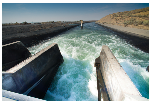
Small projects like gate modernization and meters are examples of projects funded by the Small-Scale Water Efficiency Program.
