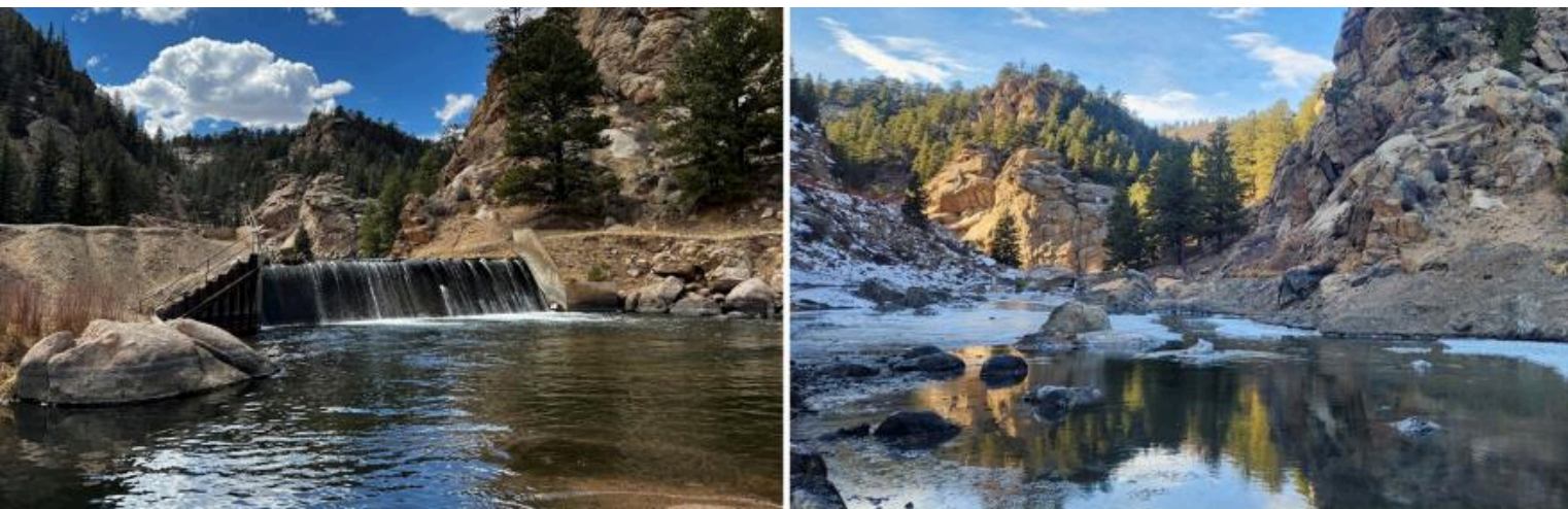
Before (left) and After (right) removal of the Lake George Diversion Dam on the Pike San Isabel National Forest. This project was funded through the first round of Collaborative Aquatic Landscape Restoration Program funding. Before removal, the dam was a barrier to movement of aquatic species throughout the system. (Credit:, USDA Forest Service)
