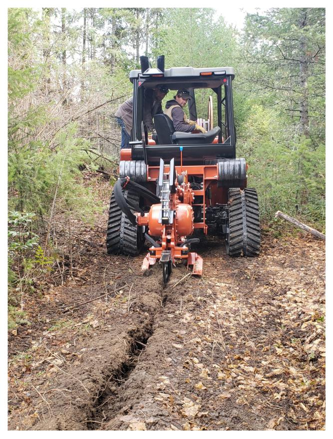
This vibratory cable plow is used to install underground distribution circuits, serving rural communities in Ferry and Okanogan counties
