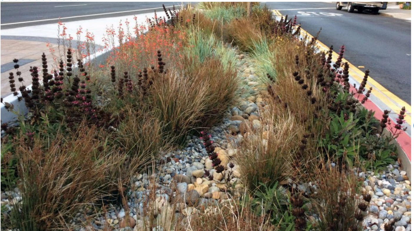
Bioswale reduces polluted stormwater runoff along Cesar Chavez Street in San Francisco, 2014. Photo: Ananda Hirsch.
