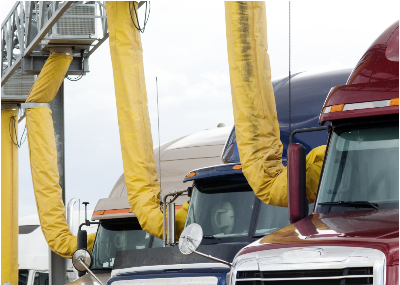
Example of a Truck Stop Electrification installation (an auxiliary HVAC unit) to reduce truck idling for cooling/heating.
