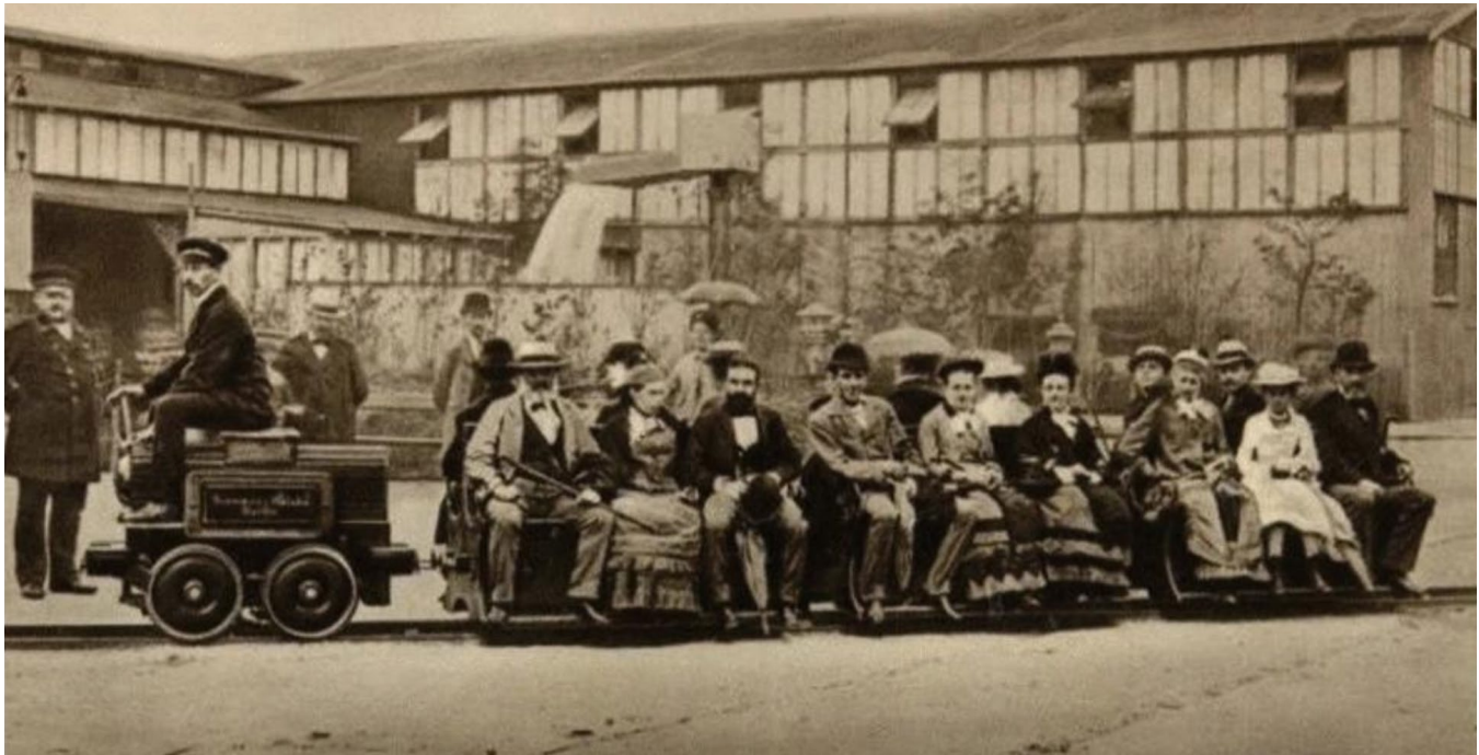
Figure 7: First third-rail electric locomotive, World Trade Fair, Berlin, 1879 47
